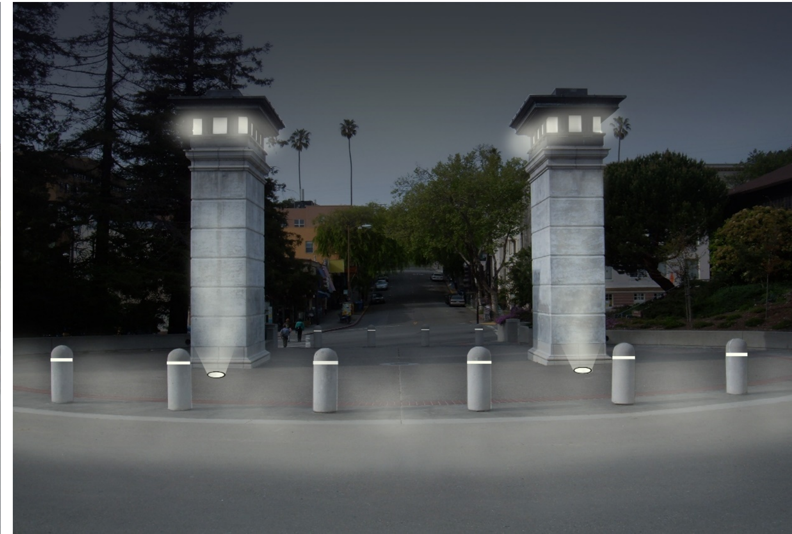
AFTER (NORTH GATE)
